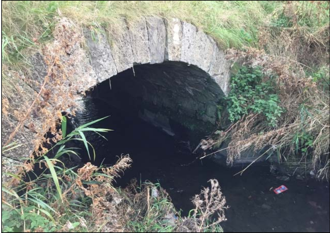
Plate 3: Onsite stone masonry bridge
