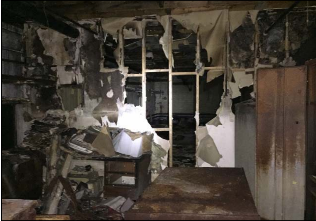
Plate 11: Vandalised interior walls
